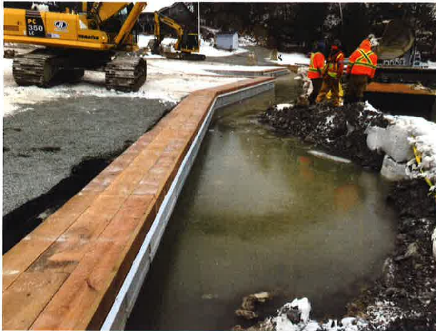
Photo 8: Progress of the Work: New retaining wall, looking west.
