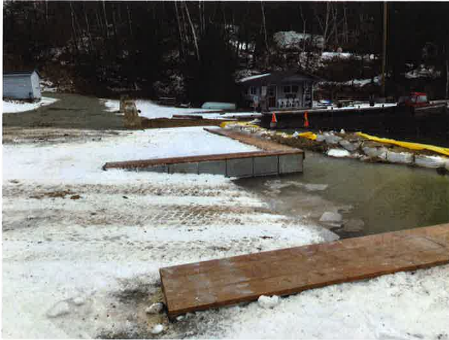
Photo 5: Progress of the Work: West section of retaining wall.
