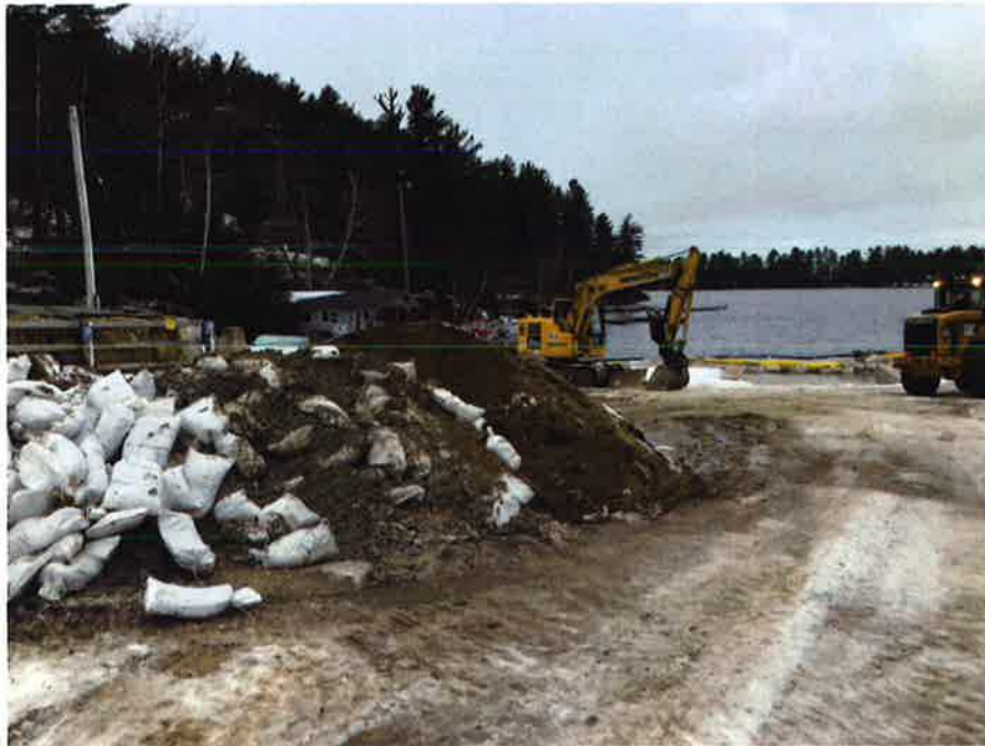
Photo 3: Progress of the Work: Sand bag removals.
