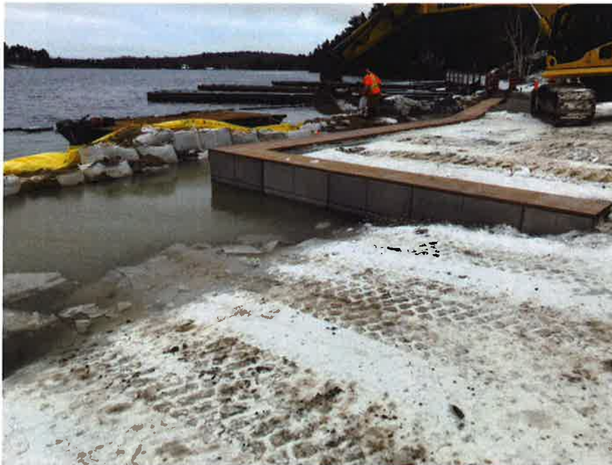
Photo 6: Progress of the Work: East retaining wall (sandbag removal in progress).
