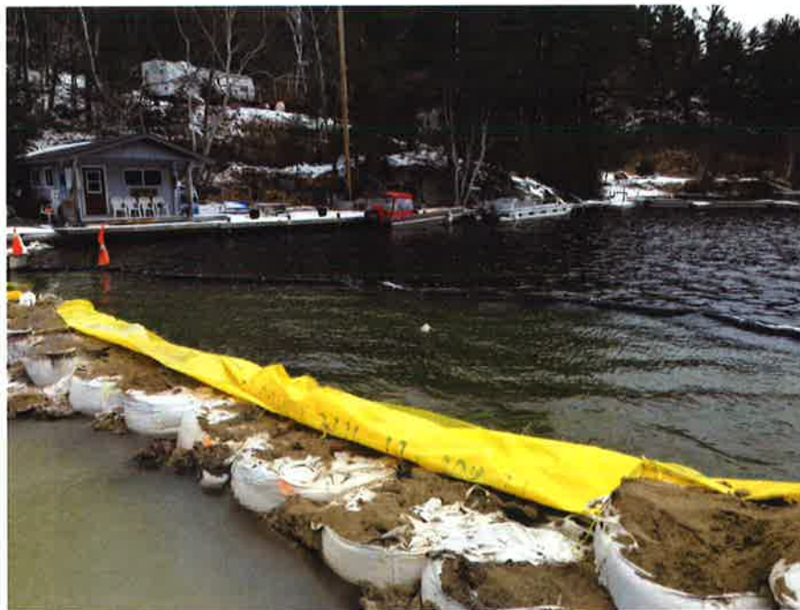
Photo 4: Progress of the Work: In-water silt curtain.
