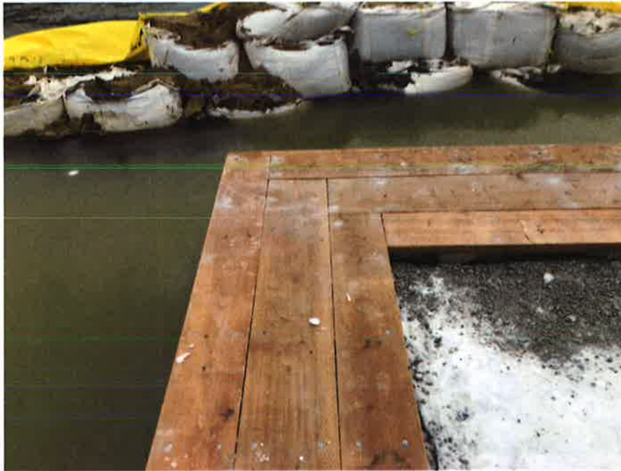
Photo 7: Progress of the Work: East wall PT wood cap.
